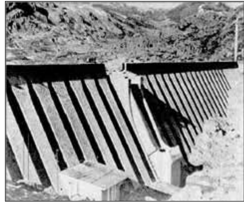
Fig. 1 Vega de Tera Dam before collapse
