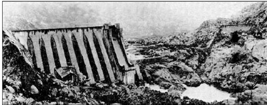
Fig. 2 Vega de Tera Dam after collapse
