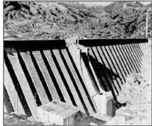
Fig. 1 Vega de Tera Dam before collapse
